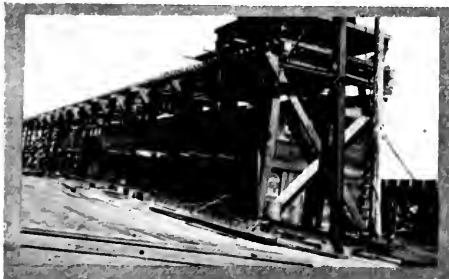
The space under the structure carrying the overhead tracks for the traveling gantry between the building berths, houses the air compressors. For further description of these pictures see the account of the plant on page 77
